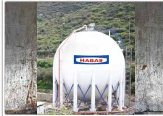
LPG tank manufacturing
